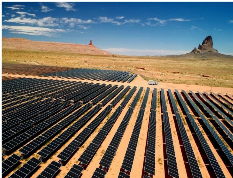
The Kayenta solar farms on the Navajo Nation, shown here in 2019, span 365 acres and produce 55 megawatts of power, supplying enough electricity to power 36,000 homes. Renewable energy, such as solar power, is drawing increasing attention in tribal communities as a way to build jobs for the future. (Navajo Tribal Utility Authority/Navajo Nation)
